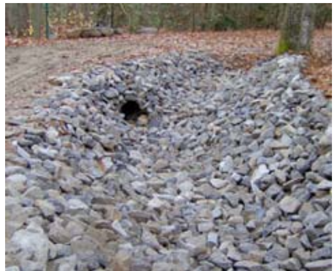
Whiting Road After Erosion Control
