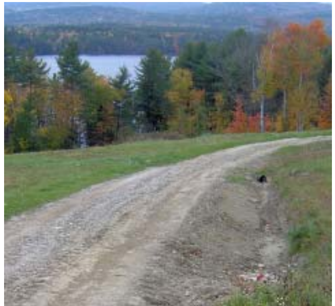
Farm Road After Erosion Control
