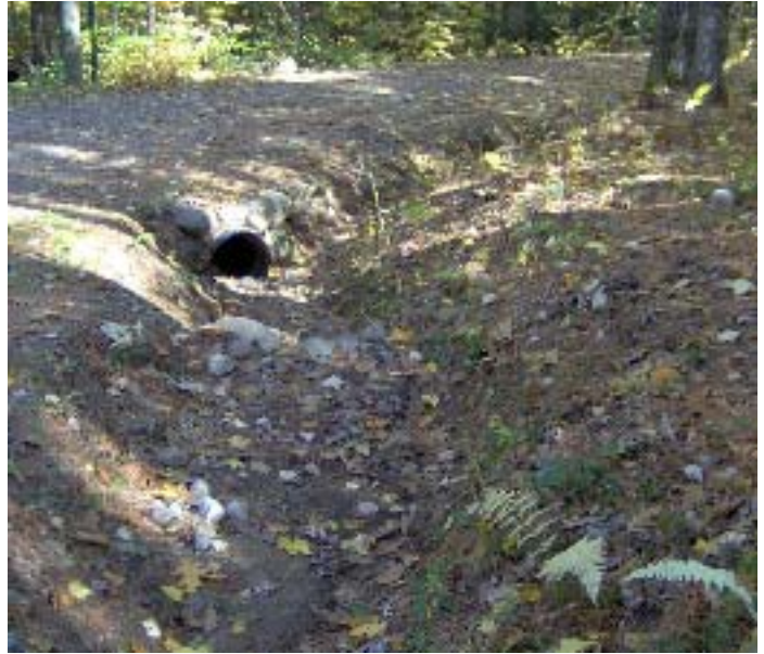
Whiting Avenue Before Erosion Control
